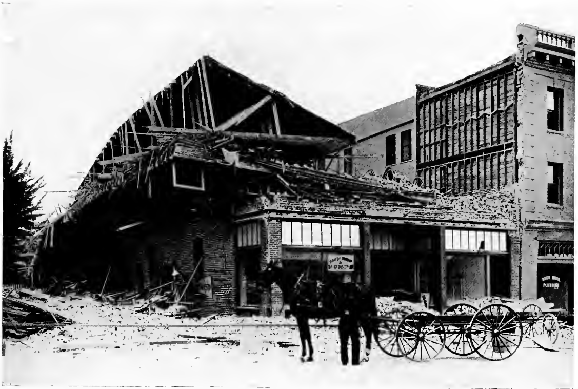
A. Wreck of 2-story brick building, San Mateo. Per J. C. B.
